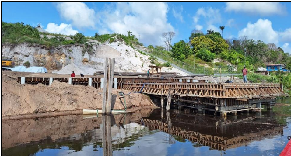
Figure 1: Wharf under construction at Tacama
